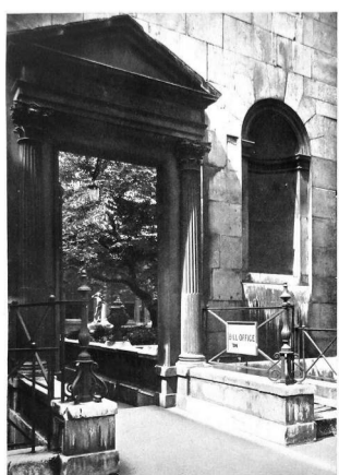
FRONT COURTYARD, WEST SIDE DETAIL OF ENTRANCE TO GARDEN COURT.
