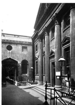
FRONT COURTYARD, NORTHWEST ANGLE.
